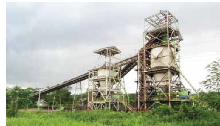
Coal conveyor belt section – KPC mine, Borneo, Indonesia, 2013.
